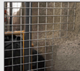
trimming around crooked walls
